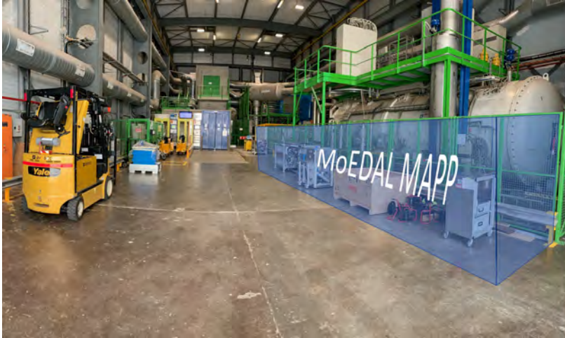
Fig. 18: The temporary staging area in SBD 2855.
