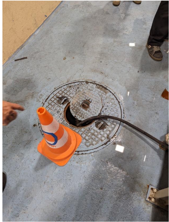
“Draining” system put in place to collect and dispose of the water.
