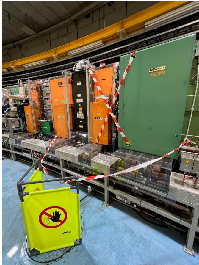
Fencing of the concerned area.
