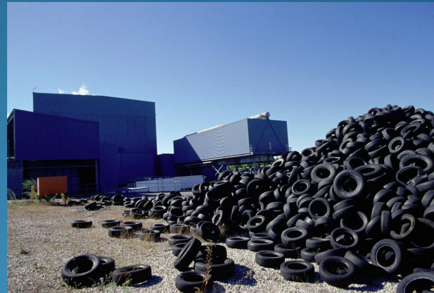
Exeter energy facility 31 MW tire-fueled power plant
