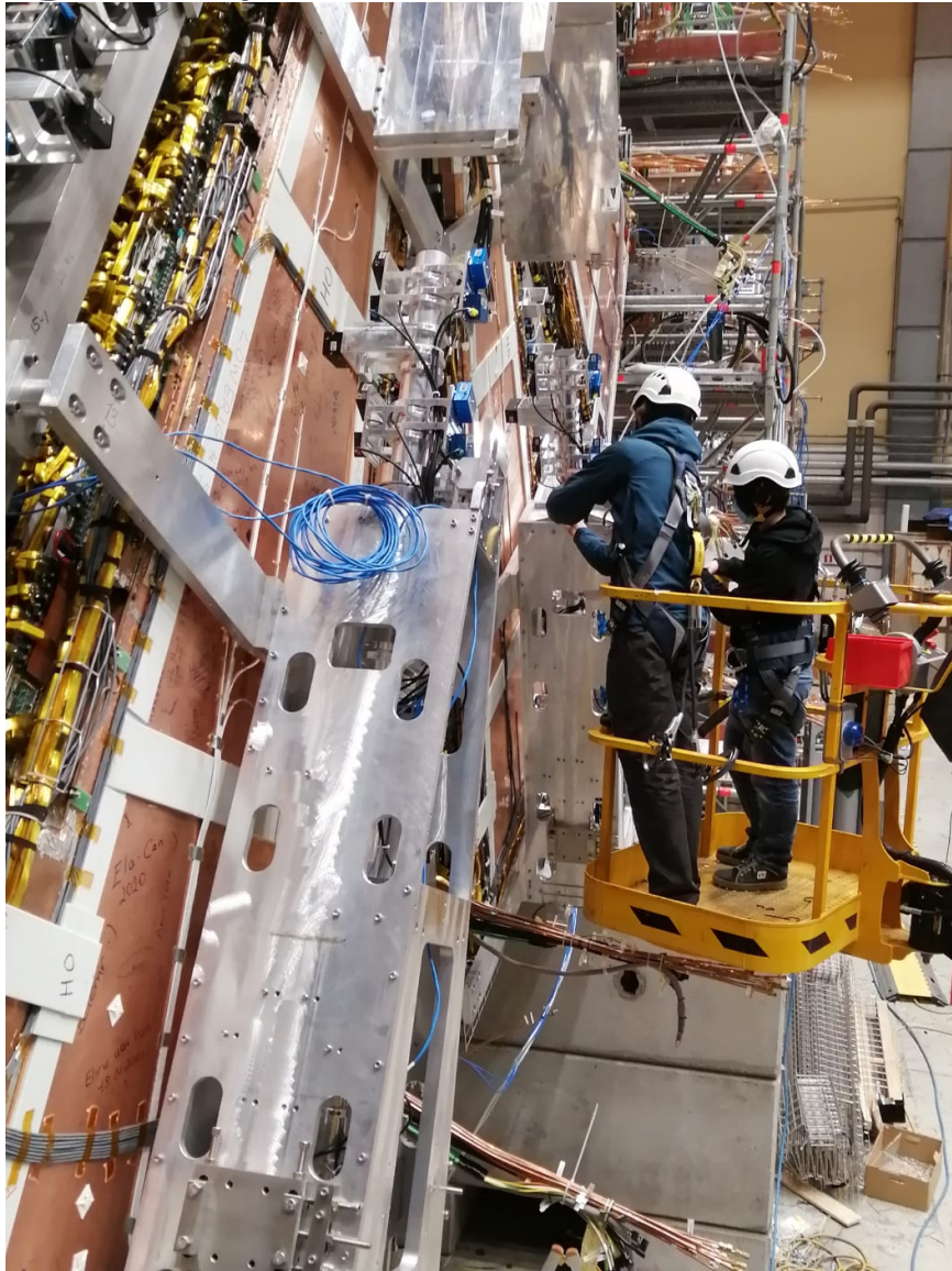
Plugging in large bars
