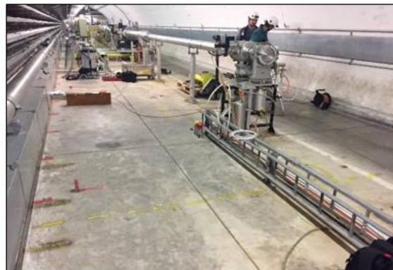
Figure 29 : Implantation and marking in SPS tunnel
