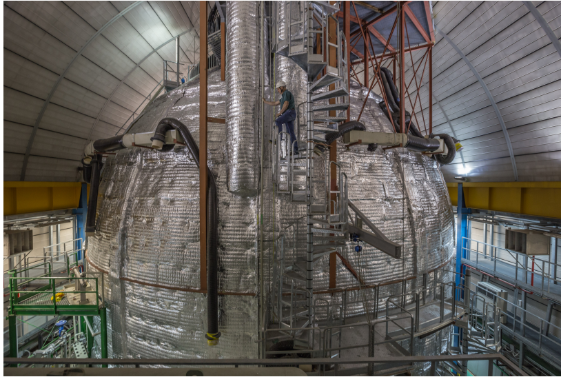
Thermal insulation of detector using mineral wool (Dec 2015)
