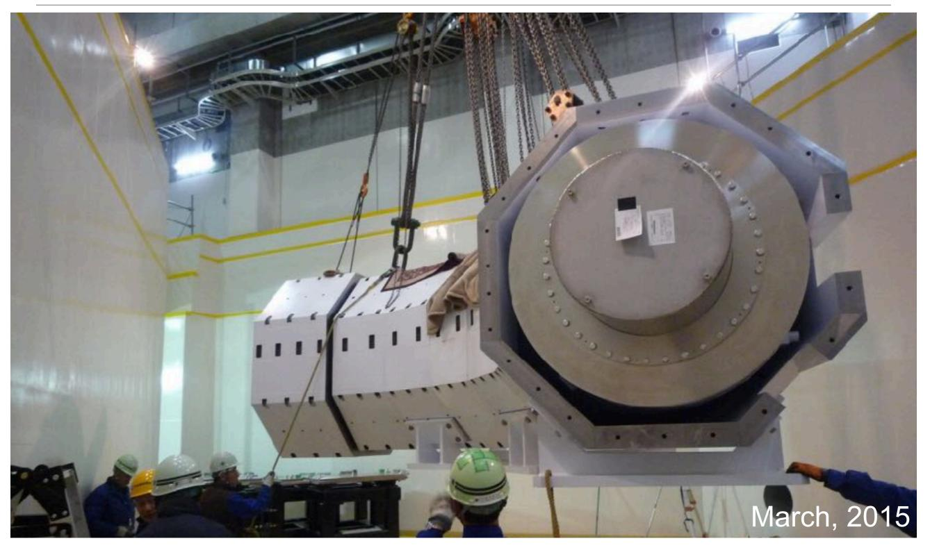
• Curved superconducting solenoid channel: ~ 3 Tesla
