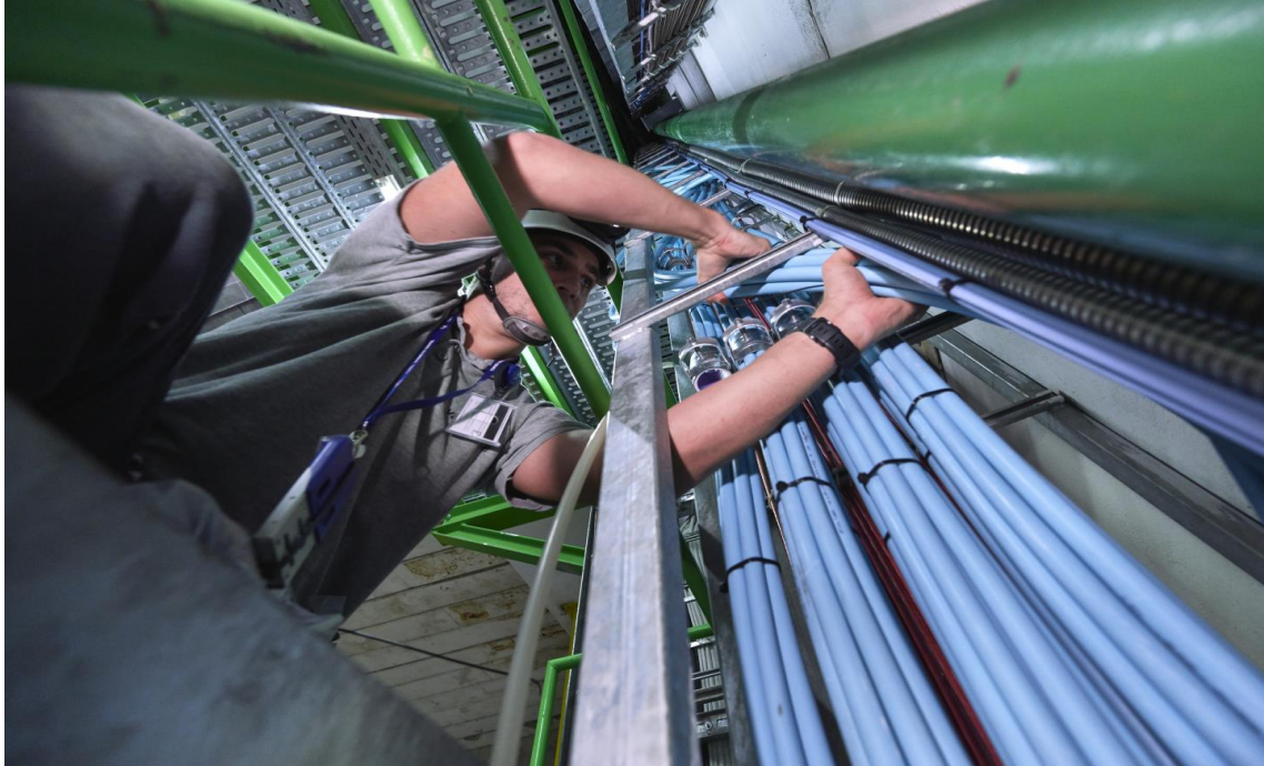
Cabling, electrical works
