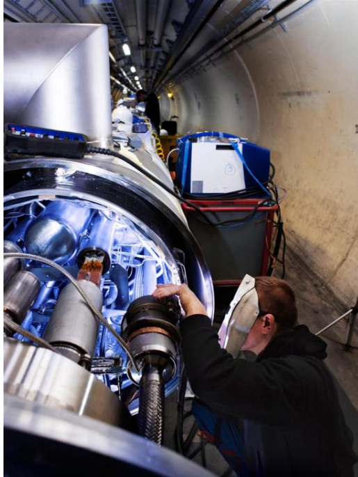
Welding and electromechanical work
