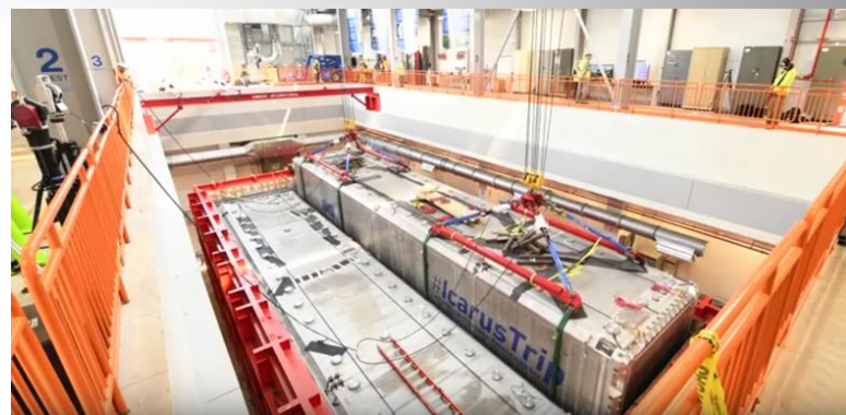
Positioning of the two ICARUS modules (cold cryostats) in final position in a new building at FNAL
