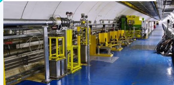
Beam test of waveguide signal
