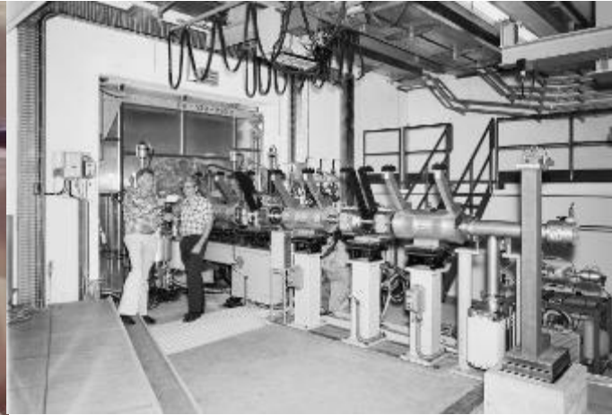
The old pre-injector at CERN (1976): Source+ Cockroft Walton +line+bunching
