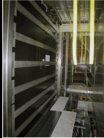
Bracing on downstream ECAL
