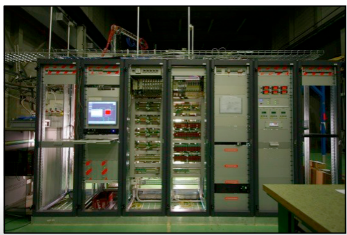
PLC-System (incl. racks for DAQ and HV) (under responsibility of CERN PH-DT group)
