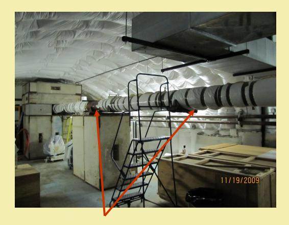
This section of beam pipe has been modified to have flanges and a bellows, so as to make it easily removable.
