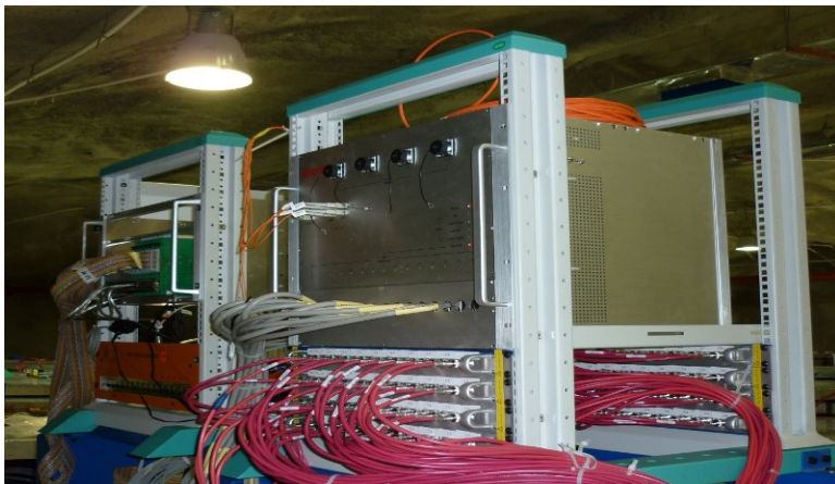
Installation of ROT
