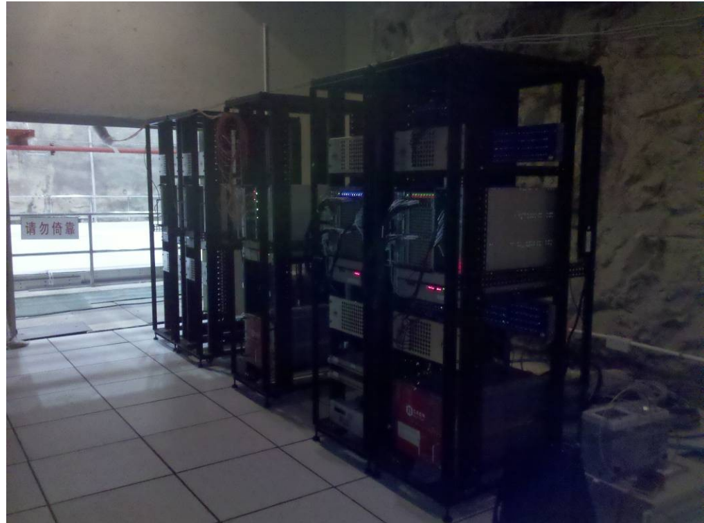
Installation and test in Daya bay Near site
