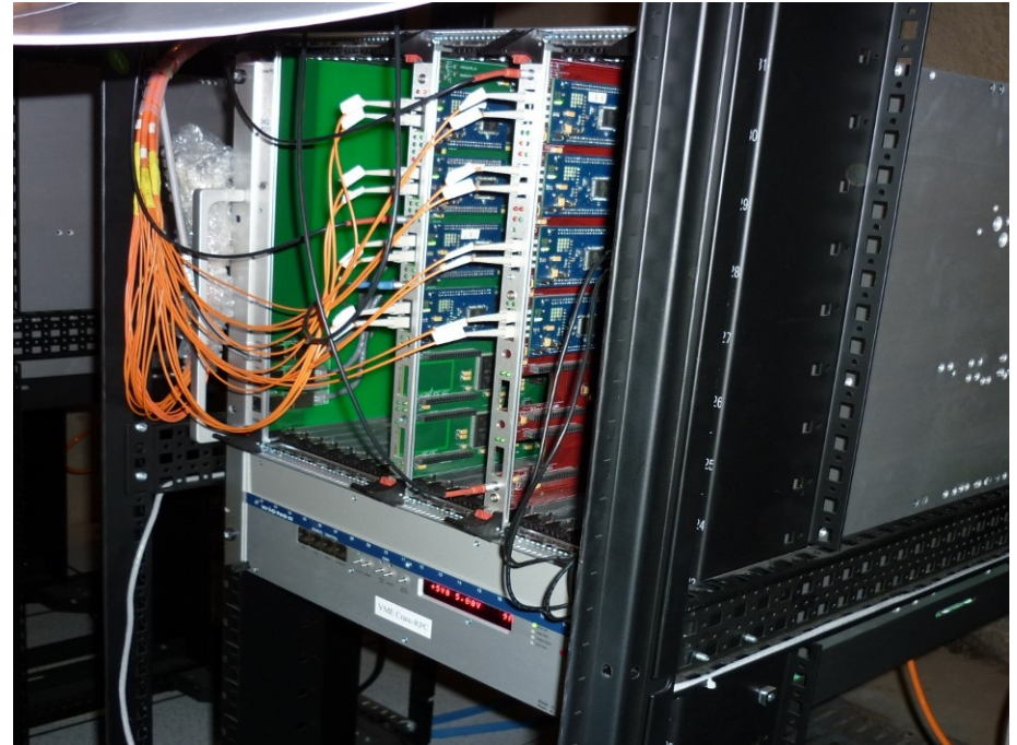
Installation of ROM and RTM
