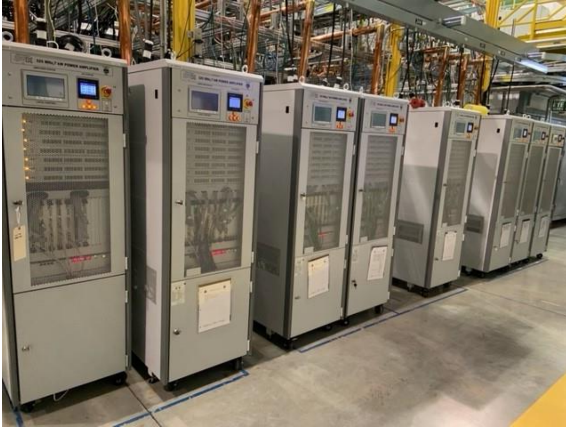
ECIL/BARC 7 kW 325 MHz amplifiers powering SSR1 cavities at PIP2IT
