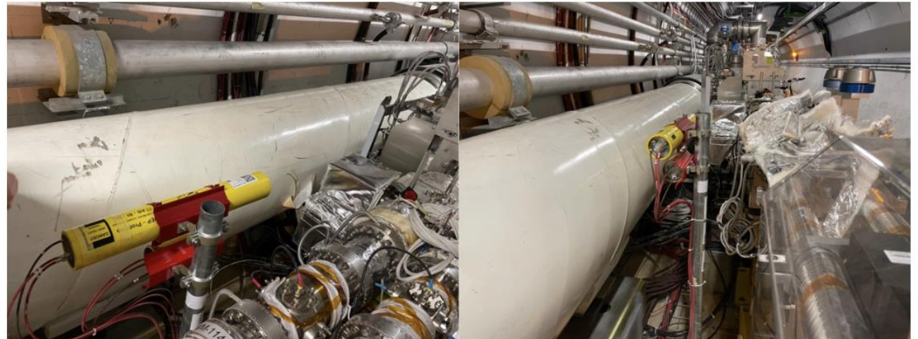
Installation in C4R8
