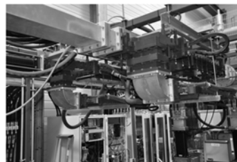
Waveguides near to klystron
