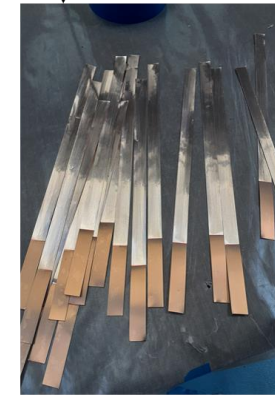
Rubbed the surface with sand paper
