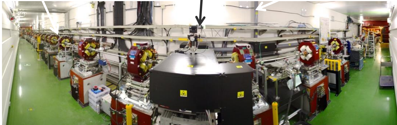
Laser beam transport
