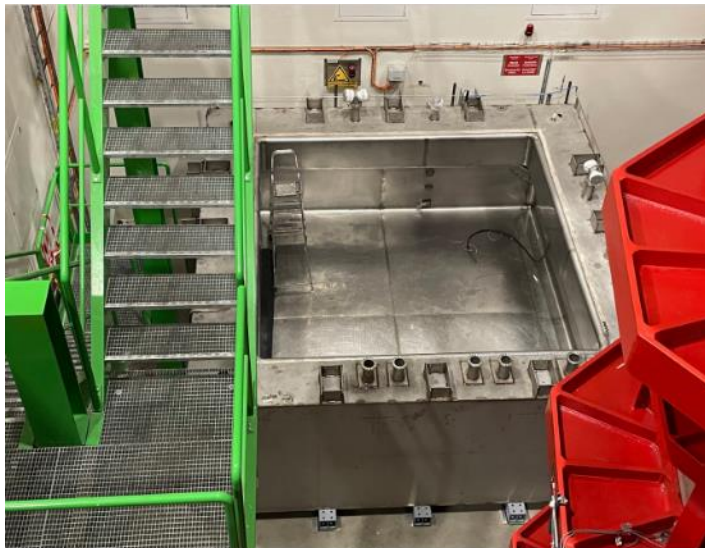
First VD Coldbox layout including rack arrangement a port assignment
