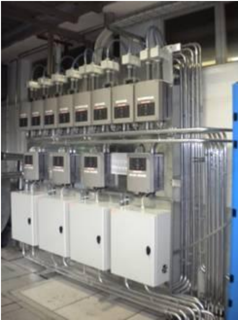
Figure 1: Air sampling smoke detectors with aspiration boxes (in this note referred as non-standard air sampling smoke detectors).
