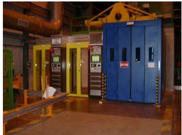
Figure 4: LHC Access System's access point. Two Personnel Access Devices (PAD) and a Material Access Device (MAD)
