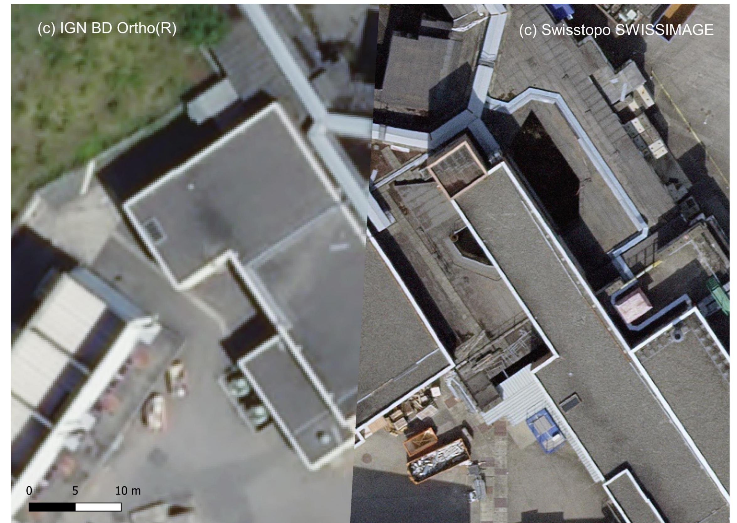
Ortophoto of the CERN Building 2002 from two different datasources
