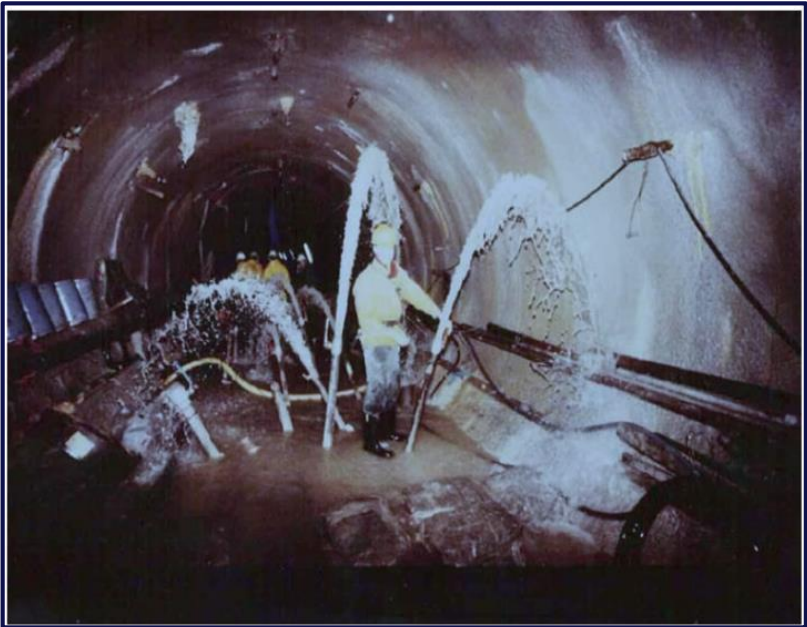
600 litres/min Water Inflow during LEP Construction
