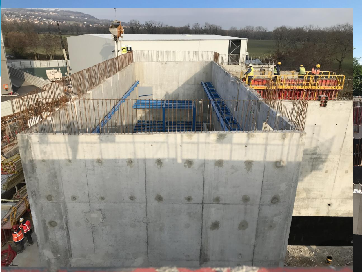
SF57: Wall casting
