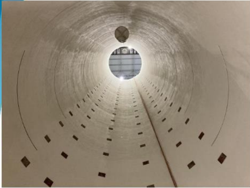
PM17 shaft final lining
