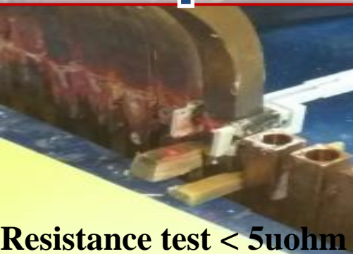
In-situ brazing of upper "C" and lower "U"
