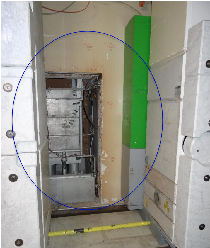
NEAR irradiation station (NEAR IN): Inside Shielding close to n_TOF target. Dedicated to R2M
