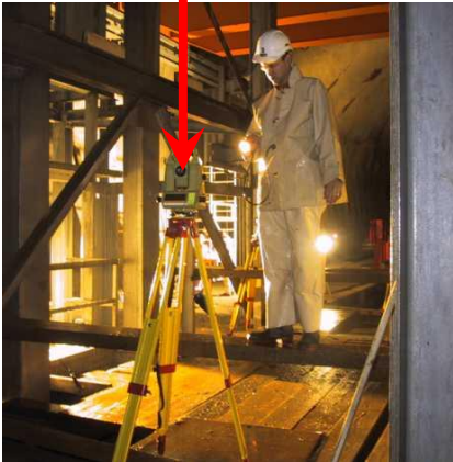
bottom of the shaft
