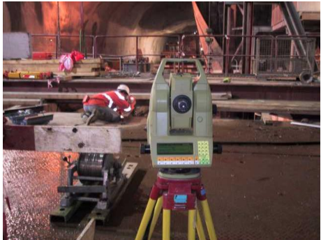
determination of the wires at the top of the shaft
