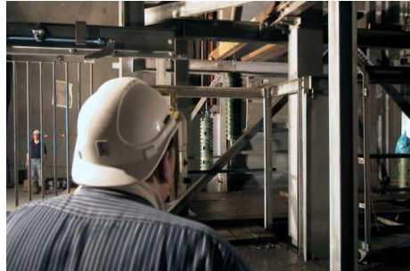
determination of the wires at the bottom of the shaft
