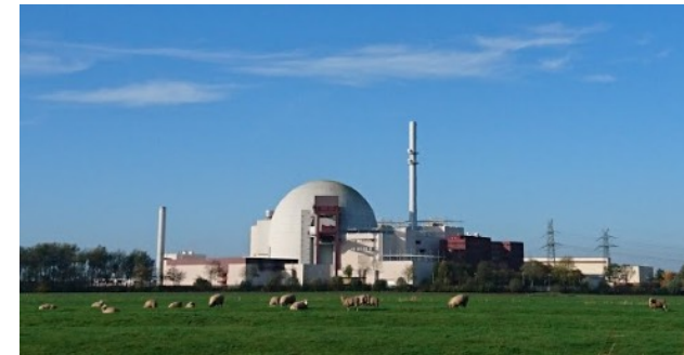
Nuclear power plant (Brokdorf, KBR)
