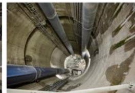
Civil engineering projects
