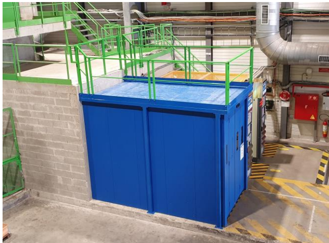
Anti-accident safety barriers installation
