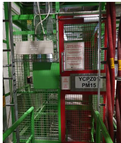
Temporary installation of control access system
