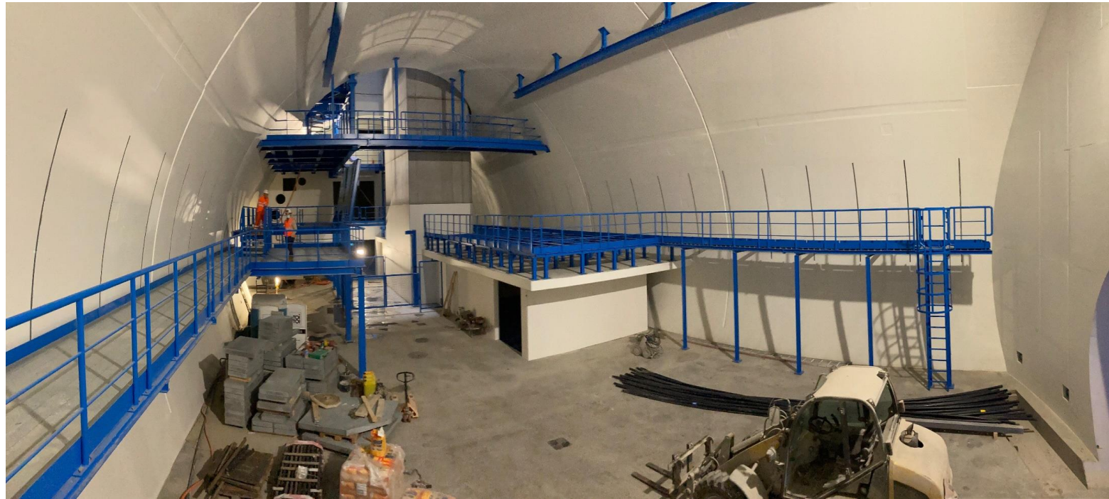
US/UW17 cavern with metallic structures for technical infrastructure
