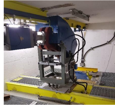
Beam delivery system
