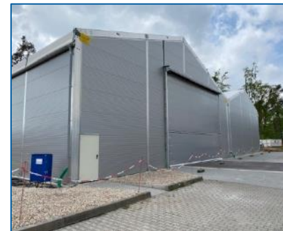
CR temporary storage facility
