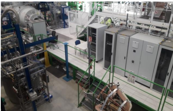
Racks for quench protection system
