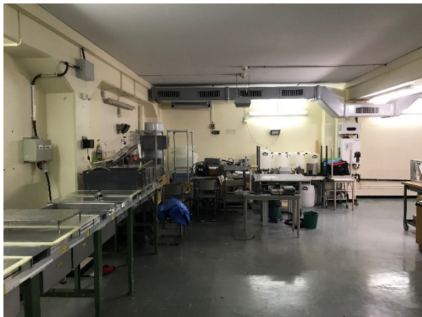
Future room for assembly
