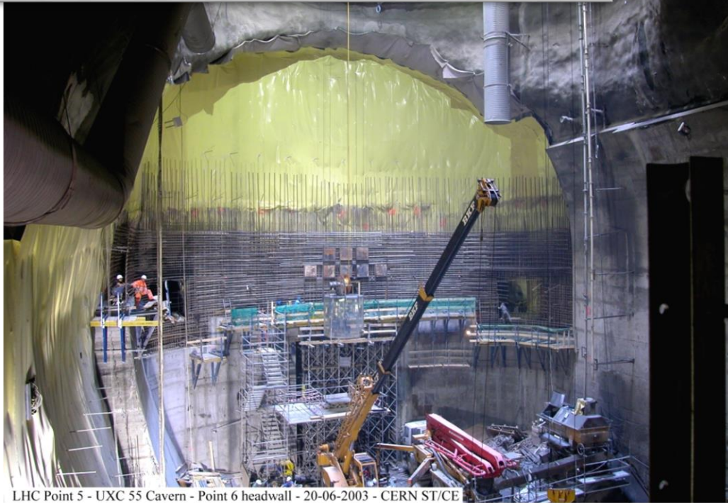
LHC Point 5 - UXC 55 Cavern - Point 6 headwall - 20-06-2003 - CERN ST/CE
