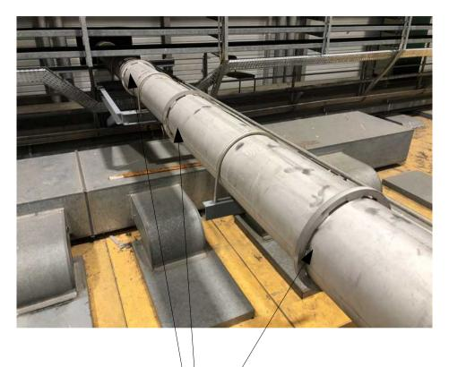
Disconnected all pipes on the concrete wall To avoid possible electronics damage by leakage current from welding
