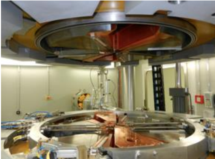
The Bern medical cyclotron and its beam transfer line.
