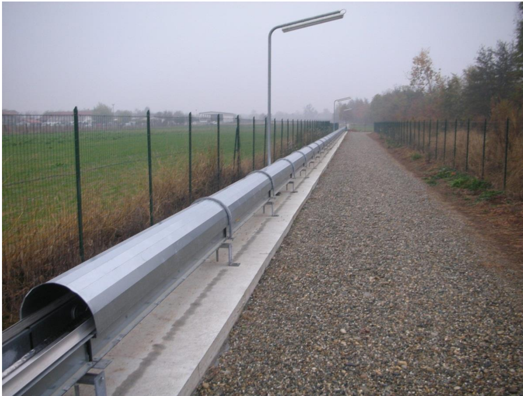
A view on the jacketing line (800 m)
