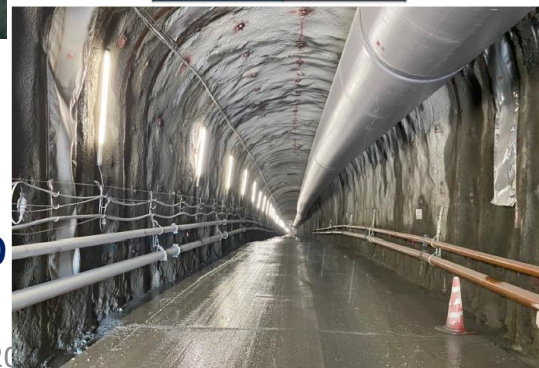
Access tunnel straight section
