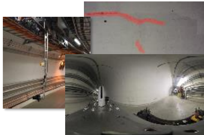
Tunnel structure monitoring
