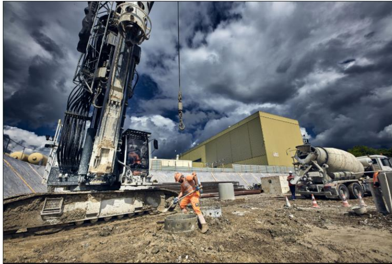
The civil engineering work for the High-Luminosity LHC gets under way. Here we see the earthmovers at work on the new 80 metre access shaft at Point 5. (Image: Julien Ordan/CERN)
