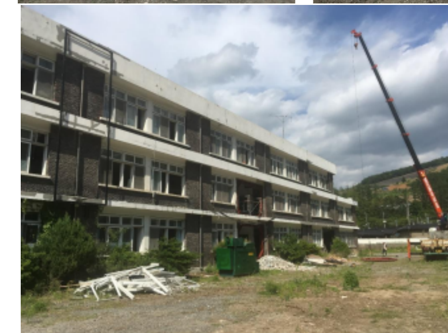
The ground office exterior
