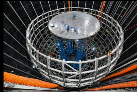
Construction progress of SS latticed shell
