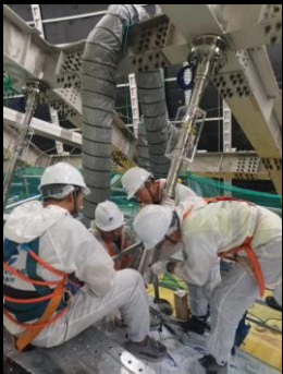
Install connection bar
