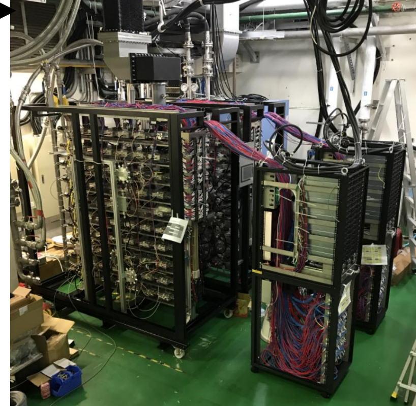
completed assembly before high power test.
