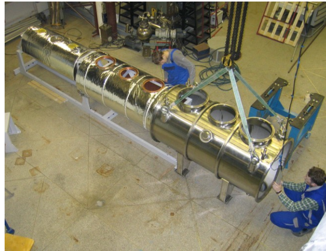
Wiggler assembling on site
