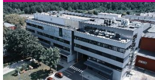
LIGHT CONVERSION SOUTH KOREA Office
