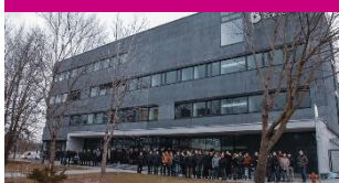
New R&D, production facilities
