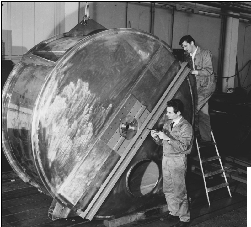
CERN PS 19 MHz Cavity (prototype 1966)
