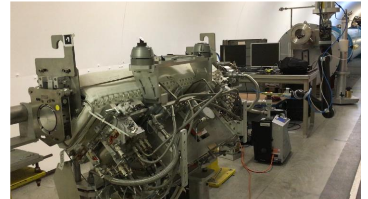
Remote Vacuum Leak detection
